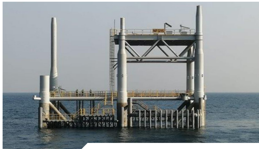
Anchored directly onto the seabed, the recently installed steel frame jackets will be used to support the deck and the topsides in fixed offshore platforms of the NFE project.
