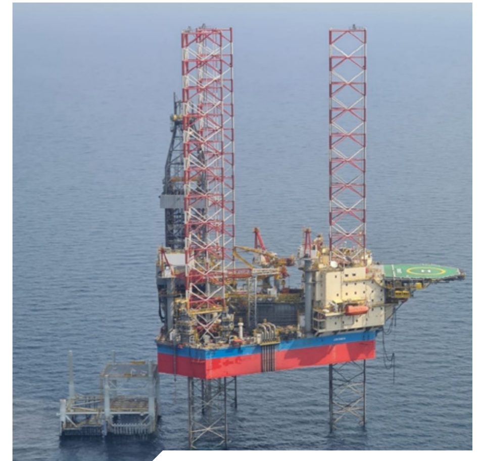
The first of 80 NFE development wells was spudded on 29 March 2020 by the jack-up rig, ‘GulfDrill Lovanda’.
