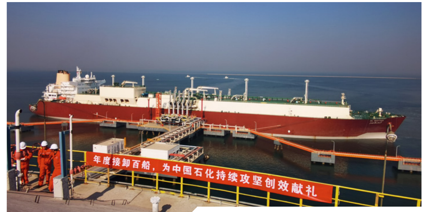
Qatargas Q-Max LNG carrier 'Al Mafyar' delivering its cargo to the Tianjin terminal, which has a capacity of six million tonnes per annum (MTPA) and is currently being expanded to handle up to 10.8 MTPA by 2022.
